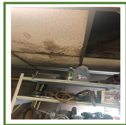
Photo 52: Roof Leak
