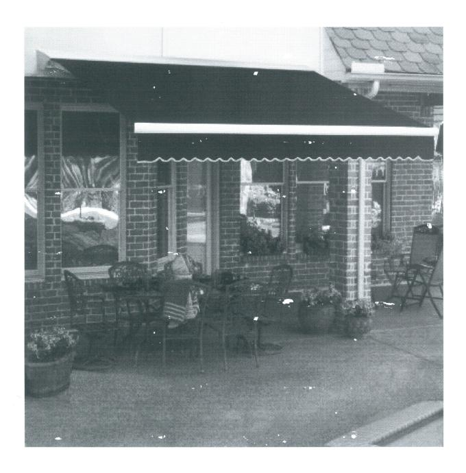
Sample of Projection and Look. Awnings are attached to the building and will be manually extended. Awnings are 15.5 wide and fully extended project 10′ 3″. They will be mounted on the left and the right of the entrance.
