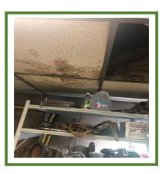
Photo 52: Roof Leak
