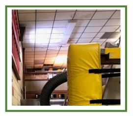
Photo 51: Roof Leak
